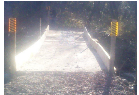
The rebuilt bridge on S70 near Joslyn School Rd.
